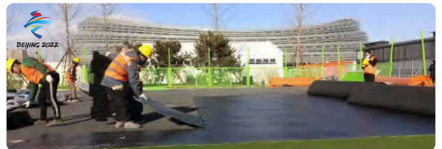
AVG artificial turf non-infill system at the 2022 Winter Olympics Speed Skating Stadium
